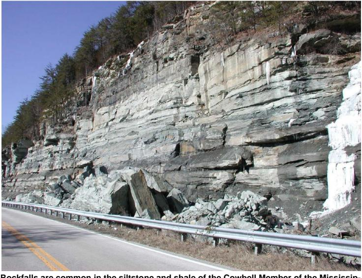
Rockfalls are common in the siltstone and shale of the Cowbell Member of the Mississippian Borden Formation along Ky. 1274 in Menifee County. Shale breaks down when wet, destabilizing the siltstone. Photo by Dan Carey, Kentucky Geological Survey.
